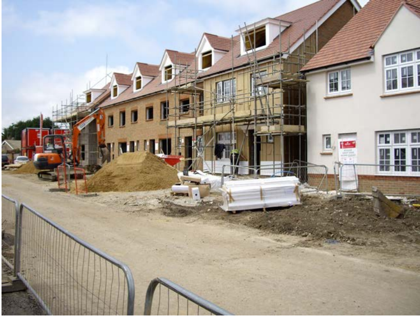
Picture 5.3.1 New house building in Faversham
