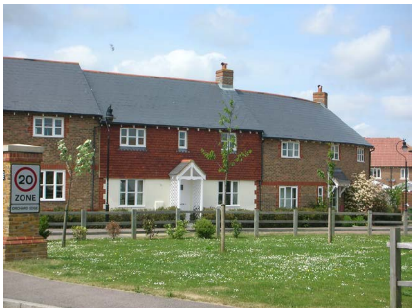
Picture 4.1.3 Good quality design and landscaping
